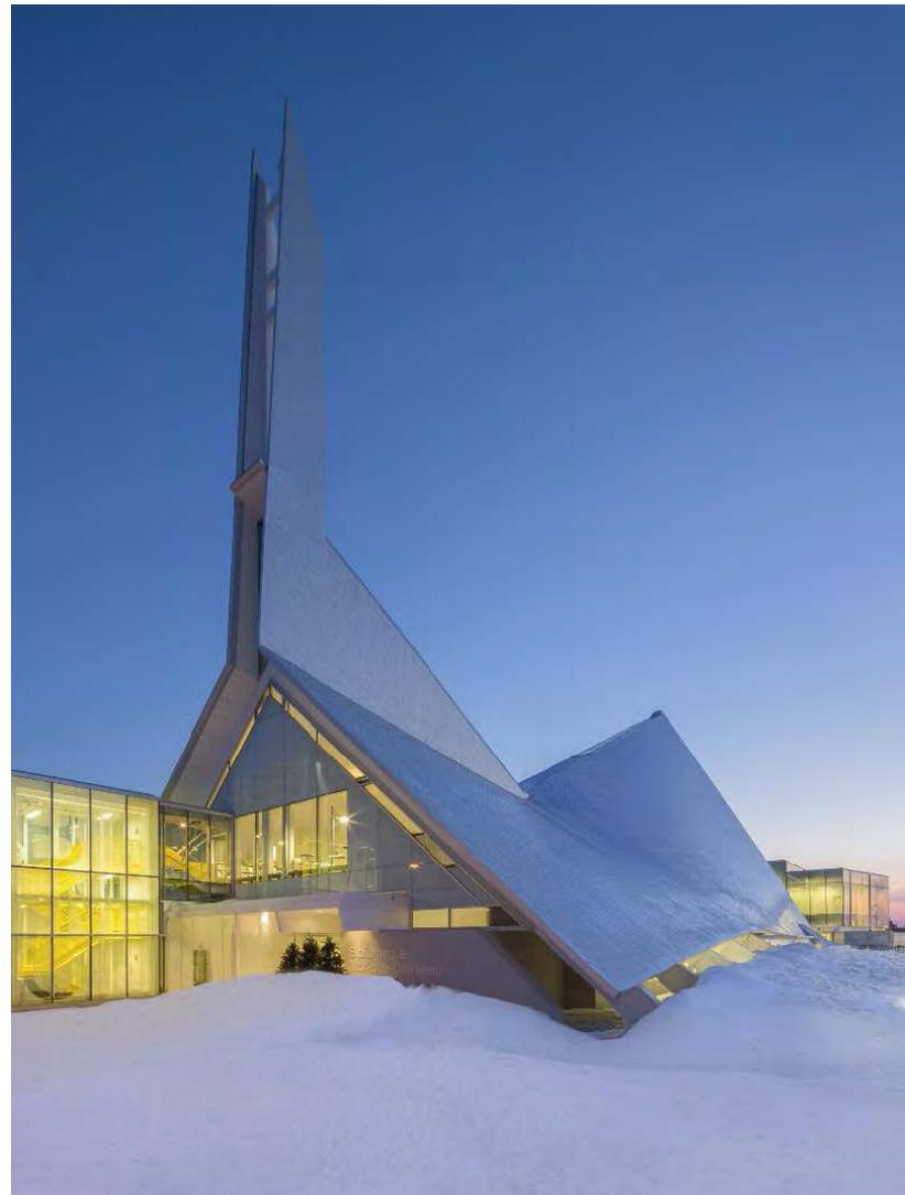
ArcelorMittal Dofasco's Galvalume Plus™ is an unpainted steel sheet product that starts with our Galvalume™ substrate and its highly corrosion resistant 55% aluminum – 45% zinc alloy hot dipped coating. A clear, organic resin coating is applied to both sides of the substrate, using sophisticated reverse roll coaters. Galvalume Plus offers strength, superior corrosion resistance and an attractive bright appearance that provides excellent heat reflectivity.
