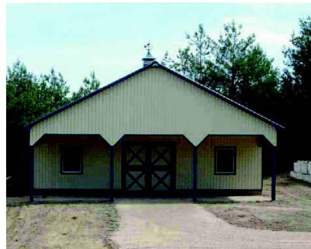
This being a high-moisture environment, ventilation is important. It is achieved here with roof vents and soft vents in the walls. Manually opened windows facilitate a crossbreeze. Walls and ceiling bear standard insulation and Super 6 vapour barrier. Moisture protection for the ceiling is achieved by means of a PVC liner panel attached to the purlins strapping the trusses.
