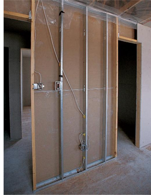
The main benefits to light steel framing are cost savings from no call-backs for warpage, nail-popping or cracks, plus ease of use.
