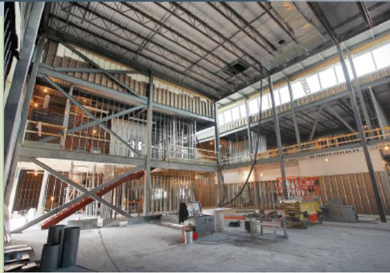
In addition to extensive use of steel roof and floor deck, light steel framing in a variety of thicknesses and sizes was used throughout the building, including wind bearing exterior walls.
