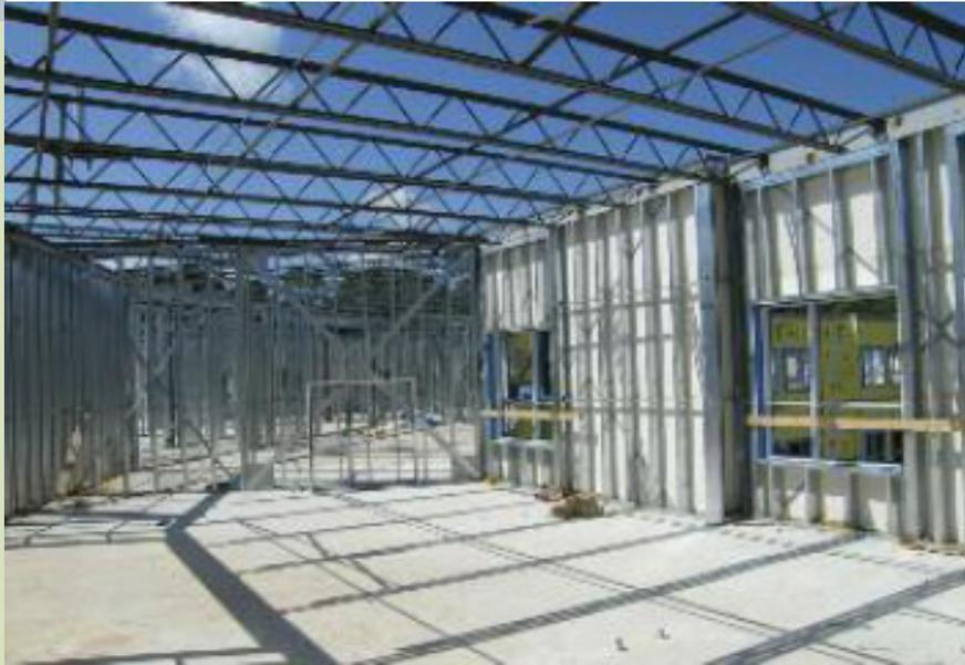
For multiple room/lodging requirements, steel is lightweight, easier to manage, requires less time to erect, does not support combustion and is totally recyclable when compared to market alternatives and, it results in less on site clutter.
