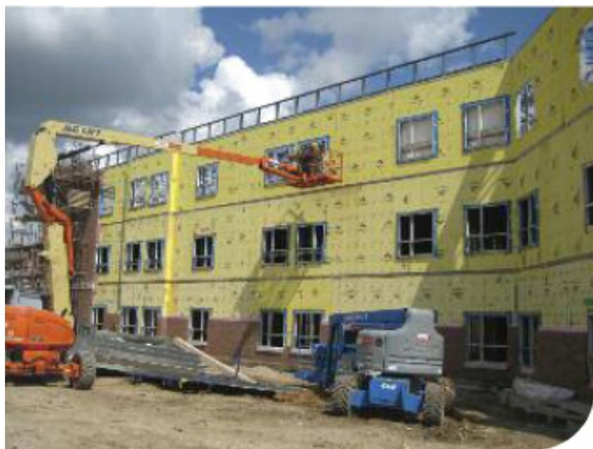
Cold formed steel wall assemblies are lightweight, strong, fire resistant and easy to manoeuvre and they allow for the structure to be closed in more quickly than competing materials.
