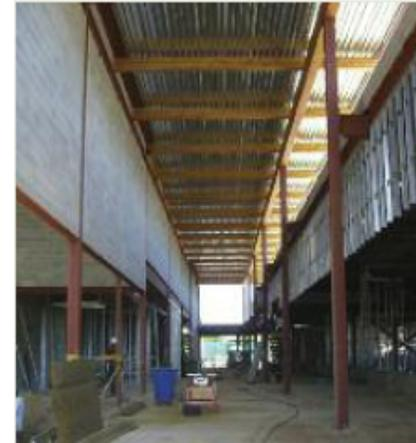
Interior of pool with finished exterior wall. The 4,422m<sup>2</sup> (47,600 sq. ft.) steel roof deck is comprised of .91mm and .61mm (.036" and .0239") ZF075 Galvanneal with 38mm and 76mm (1.5" and 3") profiles on OWSJ.
