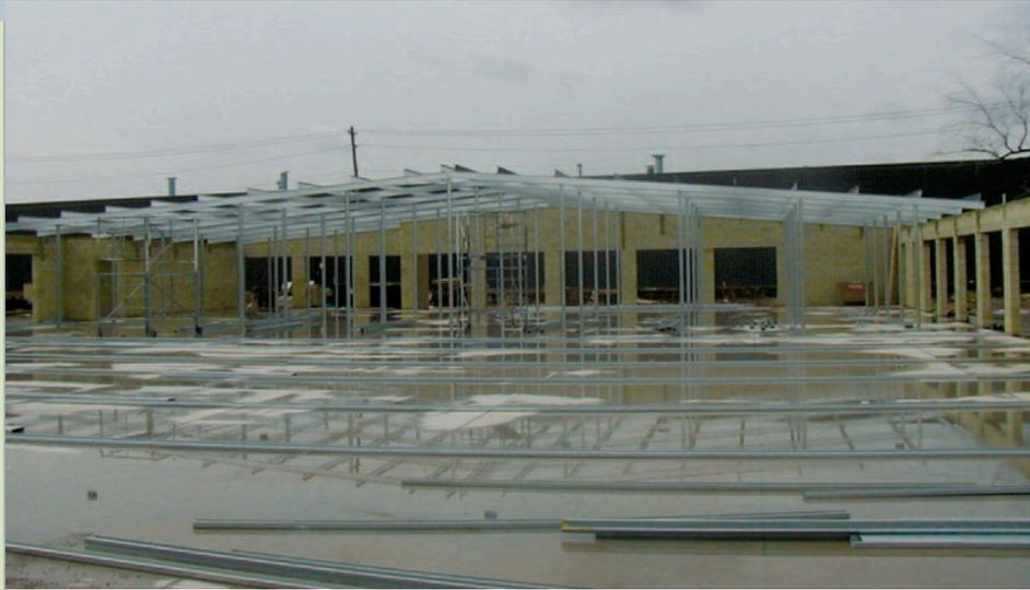
Through the use of light steel framing for the walls and less masonry construction, costs were lowered.
