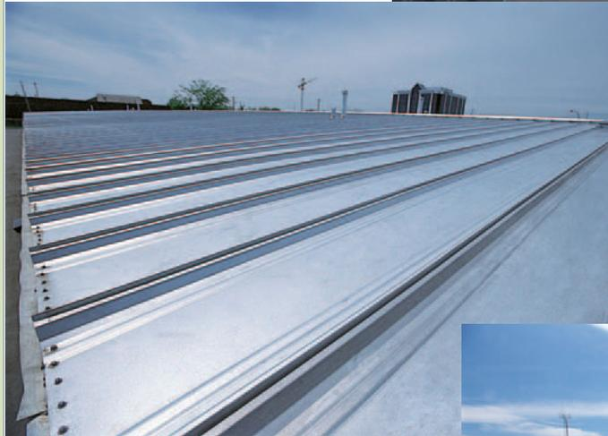
Unpainted Galvalume Plus was used for the standing seam roof. Time has proven that Galvalume steel roofs last longer, require almost no maintenance and provide exceptional value.
