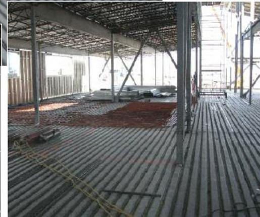
The second and main floors are concrete on a total of 3,396m<sup>2</sup> of 38mm x 0.76mm (1.5" x .0299") galvanized composite steel deck (Vicwest P-2432) supported by wide flange beam and girder systems.
