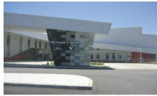
The building features sloped sidewalls, skewed end walls and the primary exterior cladding element consists of sheet steel panels. "All roof and wall cladding is prepainted Galvalume AZ150, coloured QC18783 Bright White."
