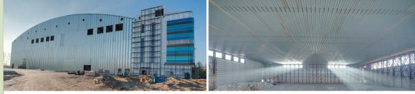
Behlen's entire panel and wall system is manufactured from heavy gauge engineered panels with an exclusive roll form corrugation that provides structural integrity. The wall system uniformly transfers the load to the foundation – eliminating expensive heavy foundations, piers and piles.
