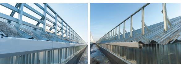
CORR-SPAN technology delivers lower energy costs due to its uniquely versatile roof system. The CORR-SPAN roof and ceiling system consists of corrugated roof and ceiling panels, joined by a lightweight, bolt together truss. The roof system provides a ventilated attic that lowers energy cost and eliminates the potential for wet insulation caused by condensation and leaks. The attic trusses can be designed for varying loads by simply changing the gauges.
