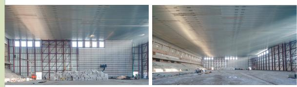
Natural ceiling, providing a bright clean interior, allows for fewer light units and lower energy bills. Natural ceiling means no exposed roof trusses, while providing a bright clean interior with high reflectivity. In this case the ceiling panels are 1.93mm (0.0758") Z275(G90) galvanized panels. The structural red iron in the photo is wind bearing.
