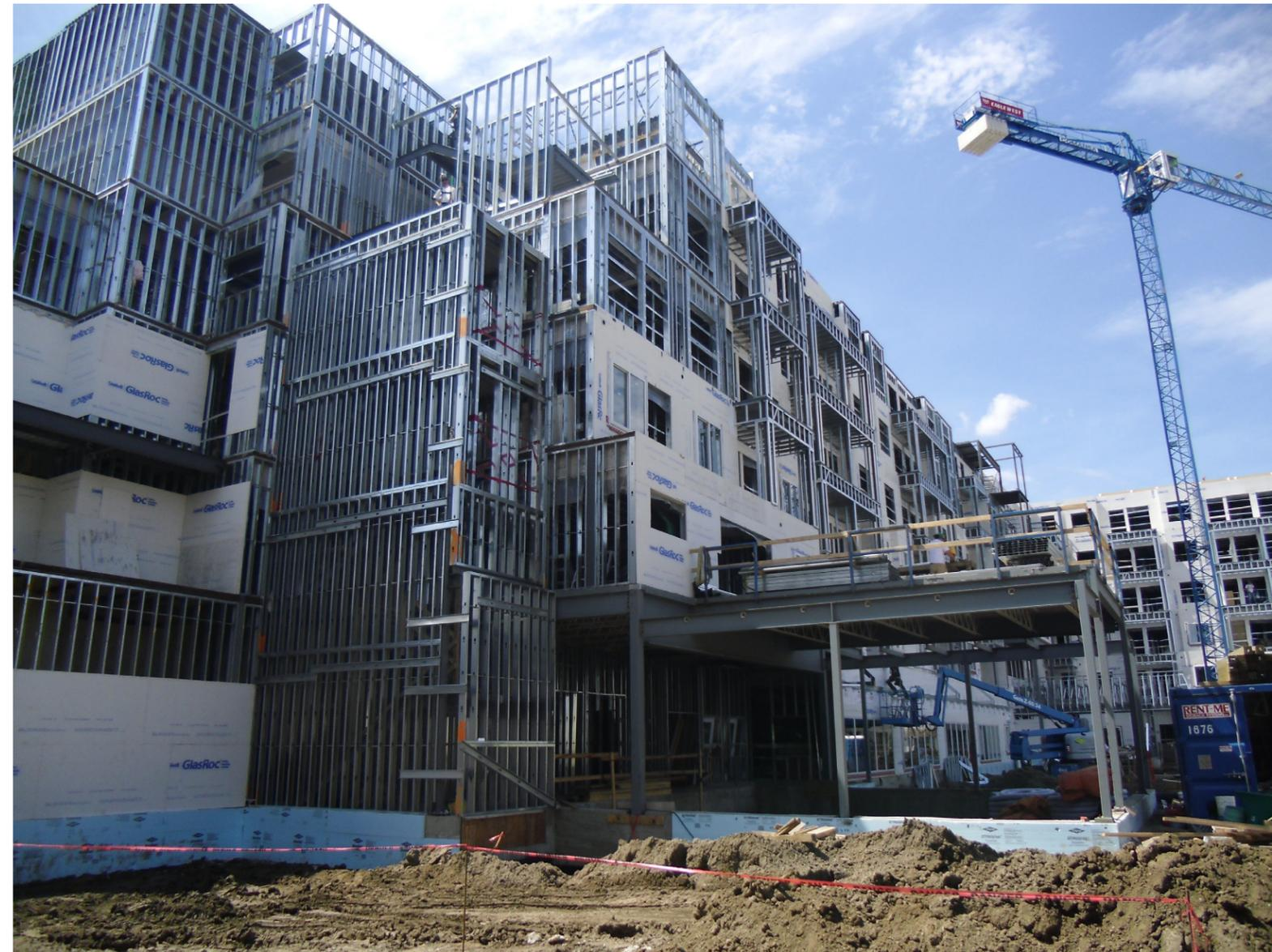
*"We supplied all the cold formed steel and connectors. We had 95% pre-cut to size to save labour and site debris. The steel's precision and straightness allowed the use of pre-engineered panels. We estimate close to a \$10.00 per 0.093m<sup>2</sup> (\$10 per sq. ft.) savings over a concrete structure."*
