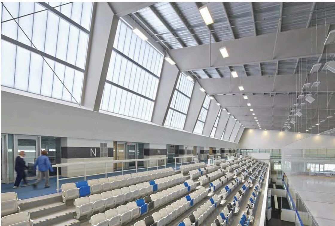
The arena building's three long span steel roofs are configured in a sawtooth pattern to provide glare-free natural light to the ice surfaces. This is achieved via north facing vertical windows of clearstory polycarbonate glazing panels.
