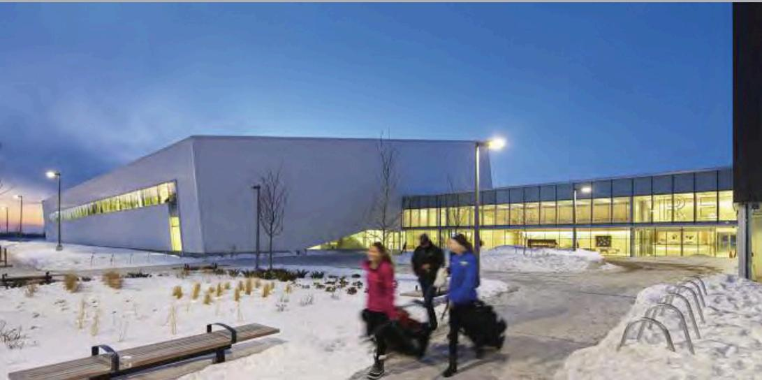
Steel was used extensively in the 15,978m<sup>2</sup> (172,000 sq. ft.) Phase 1. The overall configuration of the first phase saw two pre-engineered steel building systems arranged as parallel modular ‘program bars’ – one ‘cold’, housing three longspan arenas for ice hockey or indoor soccer – and one ‘warm’, containing the gym and library. The two buildings are connected by a conventional steel ‘link’ building.
