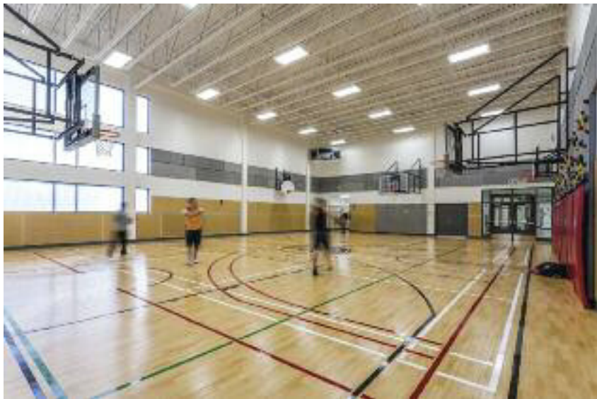
The Field House is a wide span rigid frame pre-engineered steel building. The roof of the steel building system (SBS) housing the soccer field is a "bright white" finish selected to achieve LEED heat island effect credit. The roof also utilizes Behlen's 'Thermalguard' and 'Vapourguard 32' systems.
