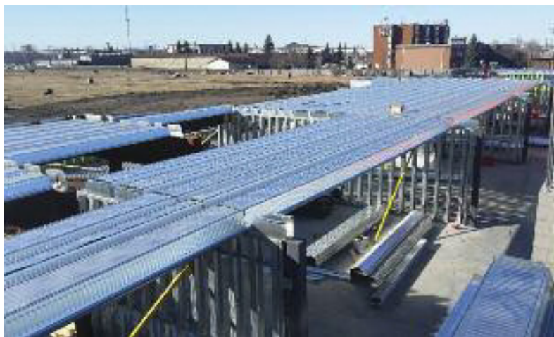
The application of the organic coating – LustreLok™ – eliminates the need for ArcelorMittal to apply conventional chemical treatment and vanishing oil. Shown in this photograph is a steel floor deck.
