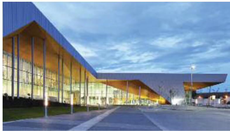
The façade is clad with .91mm (.036") pre-painted AZM275 (G90) galvanized standing seam steel cladding, coloured QC2624 Bright Silver, which begins at grade and slants upwards to form a canopy above the main entrance.
