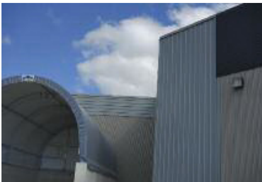
Typical Wall Section: Brick was removed, Blueskin self-adhered air and vapor barrier membrane and rigid insulation were added. Once Z bars were installed, both vertical and horizontal siding was installed, depending on the location.
