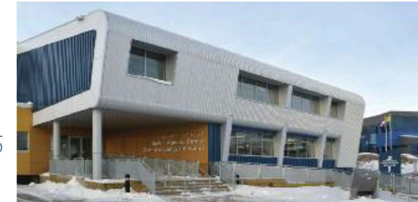
As with the Nunavut Justice Centre, shown here, in the background, Galvalume steel cladding is an integral part of the Aquatic Centre's exterior envelope.
