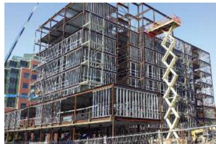
"We supplied all the cold formed steel and connectors. We had 95% pre-cut to size to save labour and site debris. The steel's precision and straightness allowed the use of pre-engineered panels. We estimate close to a \$10.00 per 0.093m<sup>2</sup> (\$10.00 per sq. ft.) savings over a concrete structure".
