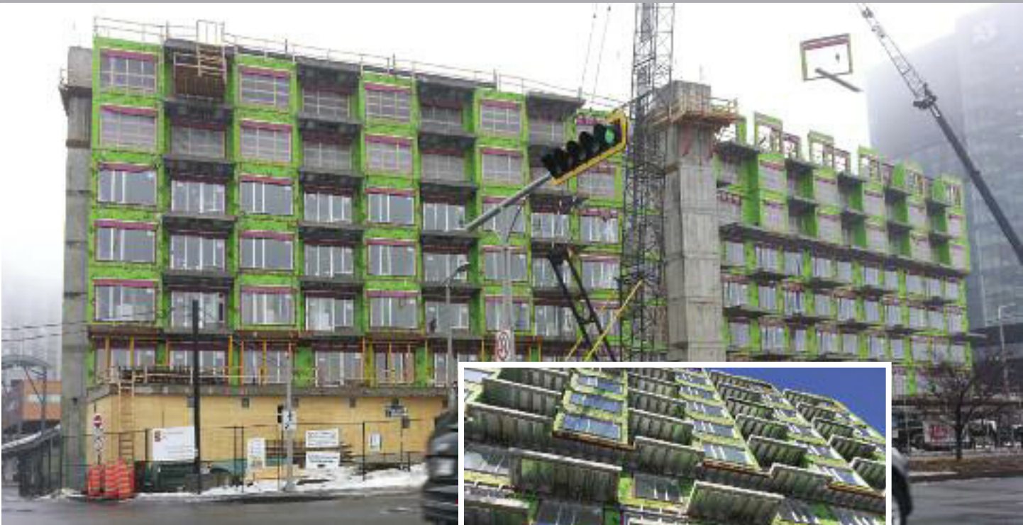
UltraBond was also used to build the balcony floors.
