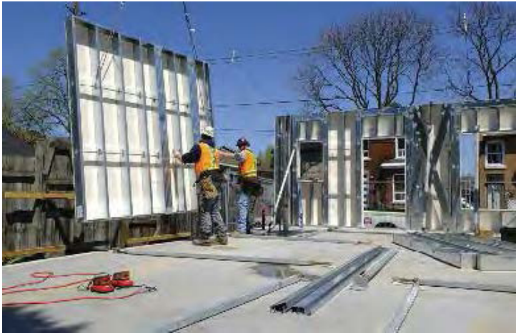
Engineered CFS wall panels are prefabricated with exceptional precision in a controlled environment, versus unpredictable field conditions. This not only guarantees a higher degree of quality, but it also prevents unexpected schedule delays due to weather conditions and other factors.
