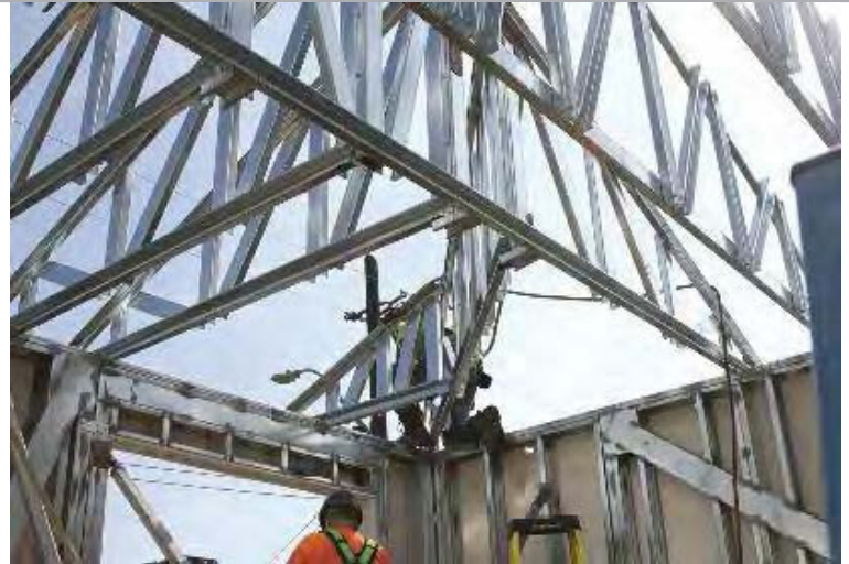
Using engineered prefabricated CFS wall panels, pre-assembled roof trusses and selected floor systems Interbuild can complete your project in a fraction of the time needed for wood/concrete frames, resulting in faster on-site erection, minimal on-site wastage as well as savings in on-site storage space of raw materials.
