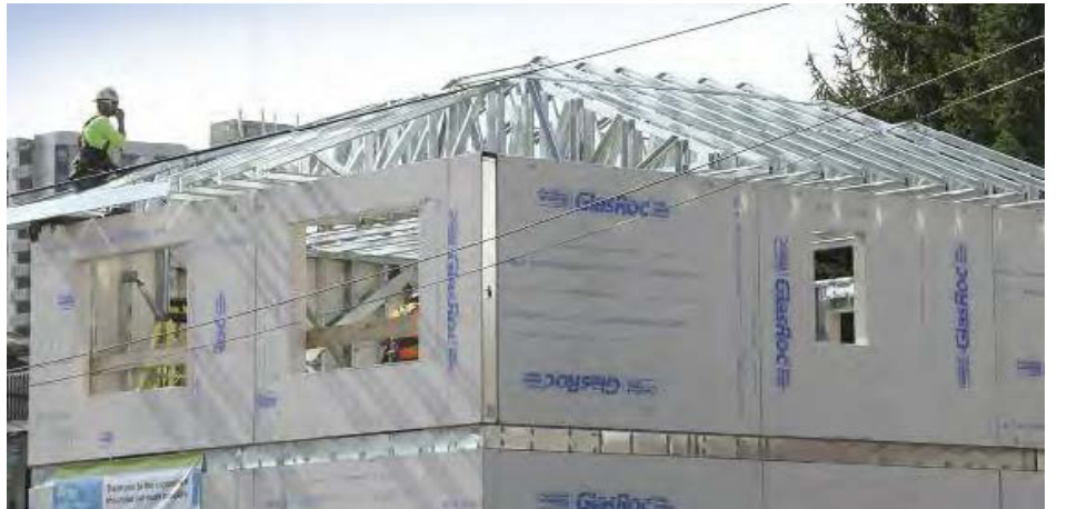
Interior view showing prefabricated roof trusses, exterior pre-assembled wall panels and interior wall studs. The floor system is comprised of a CFS panel system with a reinforced concrete overlay.
