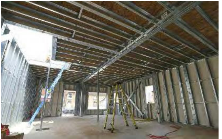
Interior view showing prefabricated roof trusses, exterior pre-assembled wall panels and interior wall studs. The floor system is comprised of a CFS panel system with a reinforced concrete overlay.
