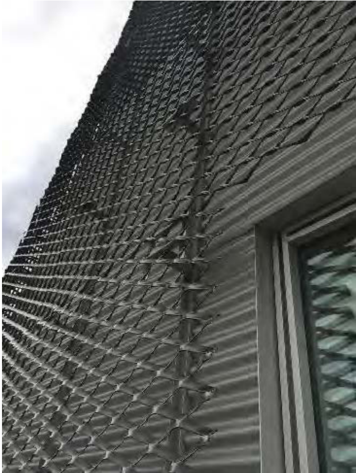
Expanded metal mesh was installed over the Galvalume.
