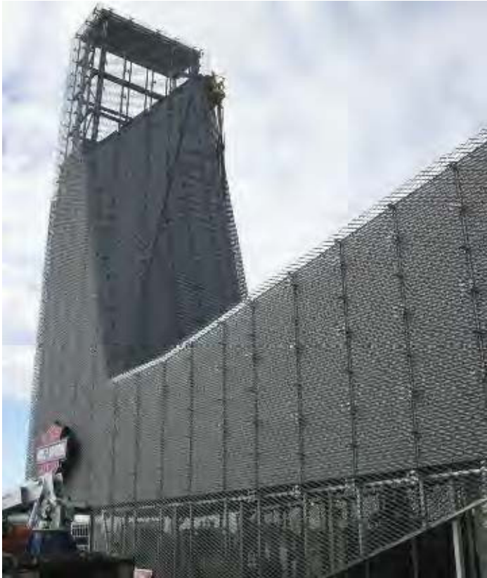
Installing the Galvalume. The top of the tower is left open.
