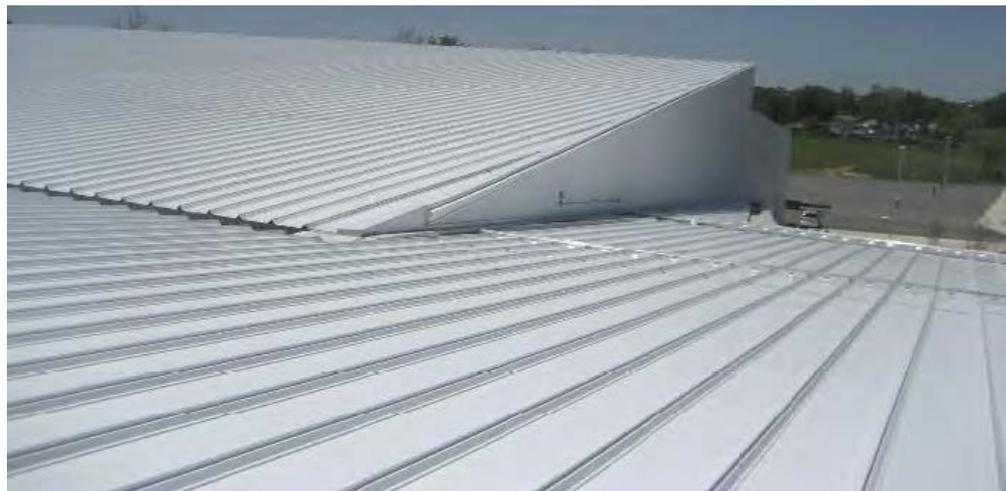
LustreLok maintains the surface appearance of galvanized steel for a longer period of time than traditional mill-applied passivation coatings and chemical treatments.
