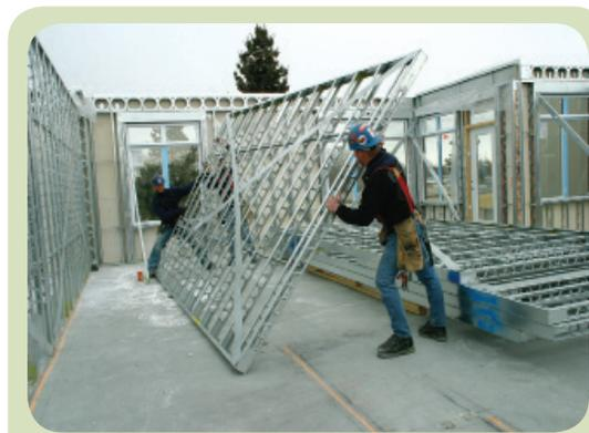
The floor joists are supported by the load bearing wall assemblies, with ZF075 galvaneal steel deck screwed down to the joists. Furring channels are attached to the joists for future attachment of drywall. Joists are spaced 609 to 1,219mm (24" to 48") depending on span and load. Mechanical and electrical services are easily installed.
