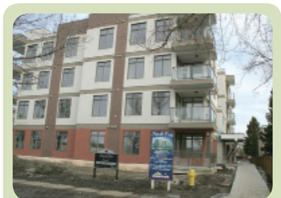
Front of the four story Park One East. The exterior load bearing EIFS envelope and interior panel assemblies were assembled in the plant and then shipped to the site. This allowed greater quality control, as well as, removing weather and scaffolding issues from the construction challenges.
