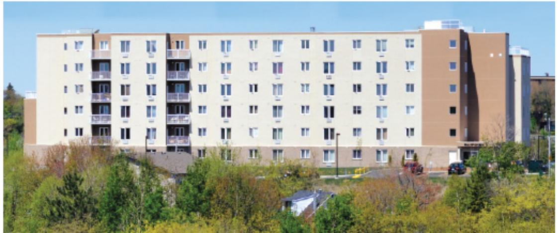
Recognizing that steel is both economical and versatile, Project Manager SalDan General Contractors Inc., of Sault Ste. Marie, decided to use light gauge steel as a complete panelized building system for the framing and walls for the Raiffeisen Co-Op Housing project. SalDan contracted Magest Building Systems Limited of Stratford, Ontario, a manufacturer of load bearing cold formed steel framing systems, to design, engineer and fabricate the 7,019m<sup>2</sup> (75,560 sq. ft.) facility.
