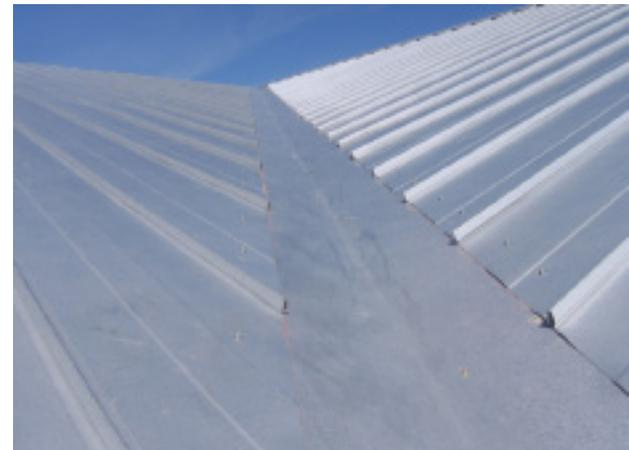
The roof is clad with the Tradition profile in unpainted .76mm (.0299"), AZM180 Galvalume Plus. The roofs of the two garages, one with a 241m<sup>2</sup> (2,594 sq. ft.) footprint, the other a 215m<sup>2</sup> (2,314 sq. ft.) footprint, are similarly clad. A total of 1,486m<sup>2</sup> (16,000 sq. ft.) of cladding covers the three roofs.
