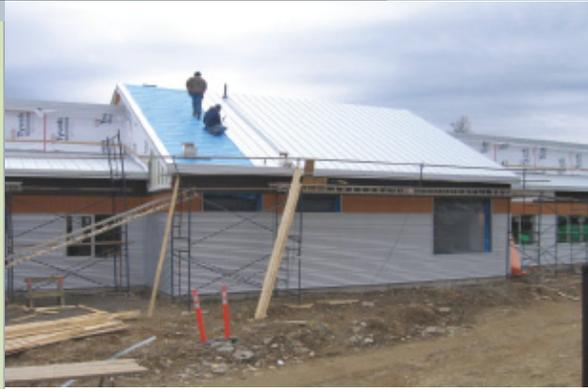
1,579m<sup>2</sup> (17,000 sq. ft.) of corrugated .61mm (.0239") prepainted AZM150 Galvalume steel cladding with a 22mm (.875") corrugated profile was used to clad the office and both garages.
