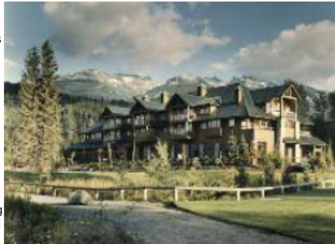
Prepainted galvanized steel was the first choice for the structure's roof from the very beginning, we knew that the roof was going to be an important design element.
