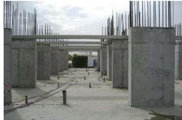
Converted ComSlab deck - bearing beams consisted of 3,352.8m (11,000 lin ft.) of 1.22mm (.048") steel. There were 54,000 lbs. (24.5 mt) of ComSlab accessories.
