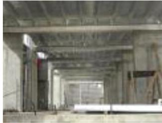
The economical benefits and effectiveness of using steel as a building material in institutional construction has long been recognized in North America and has now gained the attention of contractors in Saudi Arabia. A composite system (steel and concrete) was the choice over the conventional concrete construction method for slabs and beams. Steel plays a significant role in the design and construction for the fifteen storey, 16,258m<sup>2</sup> (175,000 sq. ft.) building.
