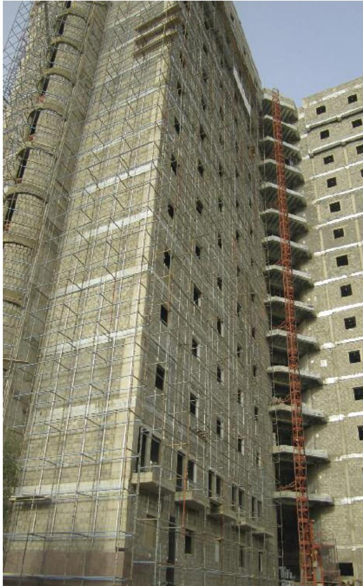
The building is one of eight being built to accommodate nursing staff at the King Fahad Medical City. The structure, which includes a rooftop skylight, was originally designed in concrete, but after a value-added proposal was presented by Bailey Metal Products, ComSlab panels and cold formed steel sections replaced the conventional concrete system for slabs and beams. The vertical columns remained as reinforced concrete.
