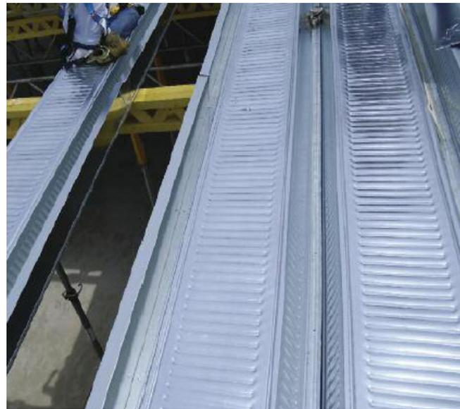
"In the new system, the beams are constructed out of several cold formed steel sections and inverted ComSlab deck, the slab and beams are poured in one single concrete pour. Forms of steel beams, inverted ComSlab deck stay in place permanently. Two steps are eliminated and, most importantly, material and time are saved."
