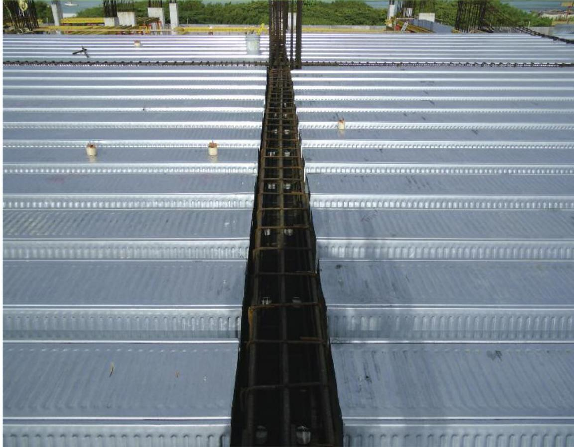
The ComSlab panels consisted of .91 mm and 1.22 mm (.036" and .048") galvanized steel with spans from 4.9m to 6.1m (16ft to 20ft). The ComSlab floor deck used .91mm (.036") steel for 12,430.6m<sup>2</sup> (133,802 sq.ft.) and 1.22mm (.048") for the remaining 3,590.8m<sup>2</sup> (38,651 sq.ft.)
