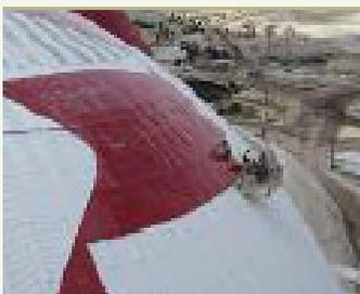
**Prepainted galvanized steel covers the copper**
