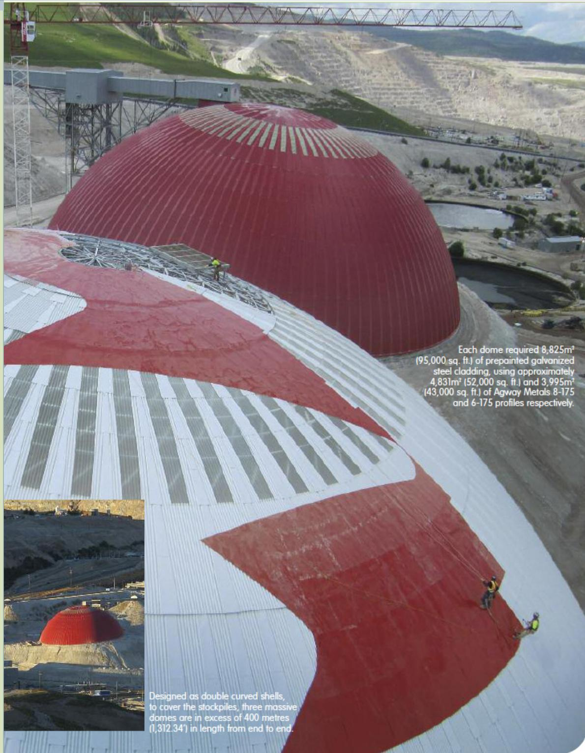
Each dome required 8,825m<sup>2</sup> (95,000 sq. ft.) of prepainted galvanized steel cladding, using approximately 4,831m<sup>2</sup> (52,000 sq. ft.) and 3,995m<sup>2</sup> (43,000 sq. ft.) of Agway Metals 8-175 and 6-175 profiles respectively.
