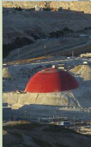
Designed as double curved shells, to cover the stockpiles, three massive domes are in excess of 400 metres (1,312.34') in length from end to end.
