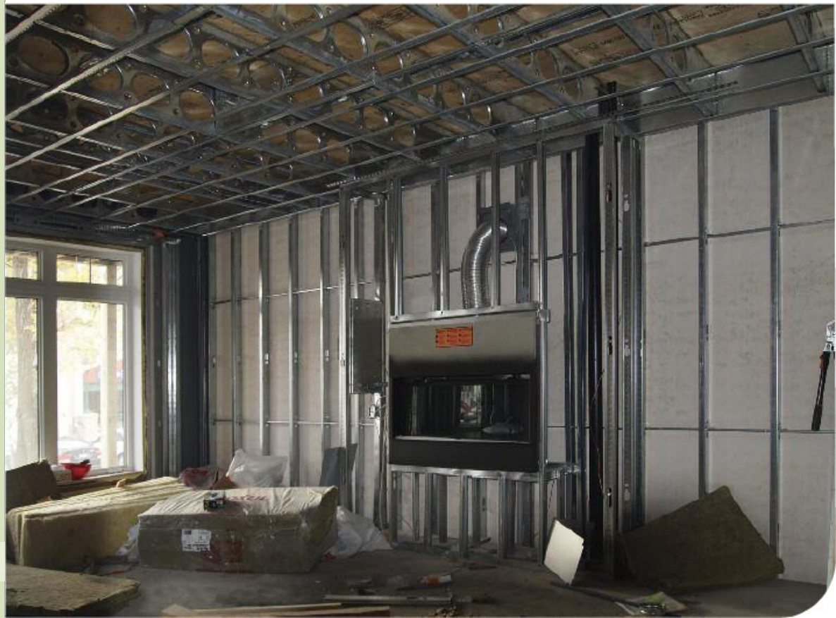
The interior of the 4,000 sq. ft. duplex is open concept with 9 foot ceilings on each floor. Since there are minimal interior walls, the steel structure had to be carefully designed to carry the load.
