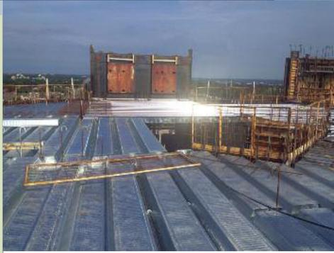
ComSlab is an alternative to the conventional concrete slab floor. You place the ComSlab, cast the concrete and the ComSlab acts as a stay-in-place form. This saves one step in the construction process and provides a cast-in-place structurally superior concrete slab.
