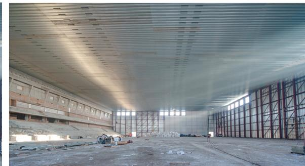
Natural ceiling, providing a bright clean interior, allows for fewer light units and lower energy bills. Natural ceiling means no exposed roof trusses, while providing a bright clean interior with high reflectivity. In this case the ceiling panels are 1.93mm (0.0758") Z275(G90) galvanized panels. The structural red iron in the photo is wind bearing.
