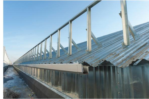
CORR-SPAN technology delivers lower energy costs due to its uniquely versatile roof system. The CORR-SPAN roof and ceiling system consists of corrugated roof and ceiling panels, joined by a lightweight, bolt together truss. The roof system provides a ventilated attic that lowers energy cost and eliminates the potential for wet insulation caused by condensation and leaks. The attic trusses can be designed for varying loads by simply changing the gauges.
