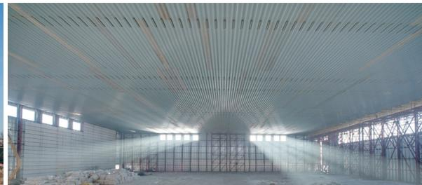
Behlen's entire panel and wall system is manufactured from heavy gauge engineered panels with an exclusive roll form corrugation that provides structural integrity. The wall system uniformly transfers the load to the foundation – eliminating expensive heavy foundations, piers and piles.
