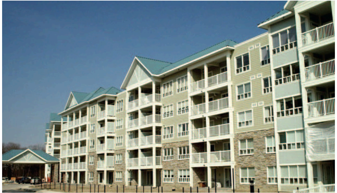
Bogart Pond Condominium Phase 1 nearing completion.
