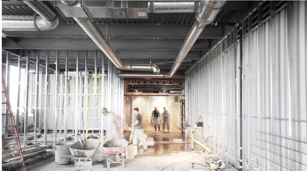
Light steel framing was selected for its noncombustible construction properties, lightweight and its ability to integrating with the new structure. Steel allowed for easily customizing all the members and elements to align with the in congruencies of the historic structure's differential grid spacing.
