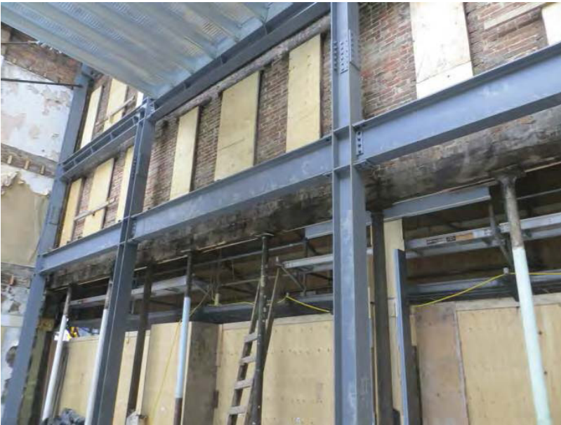
ComSlab at ground floor, ready for concrete.
