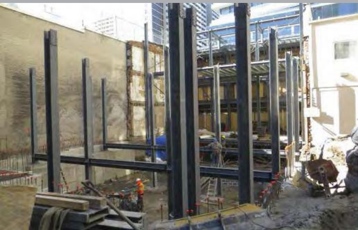
Construction of new structural steel and ComSlab.
