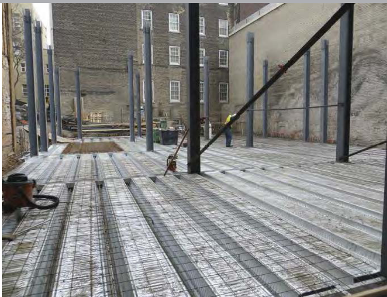
ComSlab at ground floor, ready for concrete.
