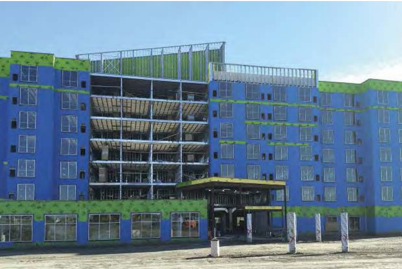
The seven-storey building comprised structural steel columns and cold-formed steel framing (CFS). It is a light weight system providing non-combustible construction, speed of installation and a faster return on investment.
