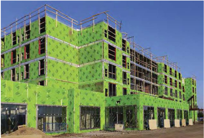
Cold formed steel wall assemblies are lightweight, strong, fire resistant, easy to maneuver and they allow for the structure to be closed in more quickly.
