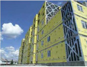
Steel, being inorganic, does not support the growth of mould nor does it give off gas, thus contributing to excellent indoor air quality.
