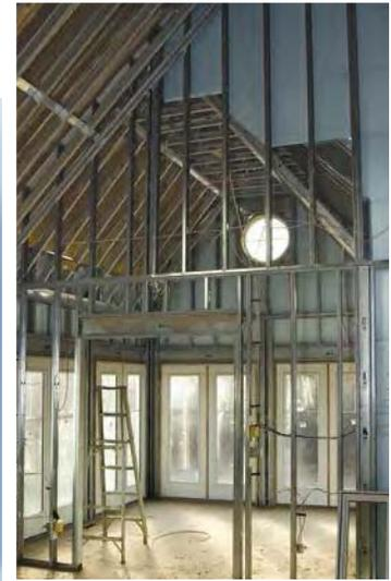
Steel makes it easier to adapt buildings to new and innovative uses. A steel building, characterized by the absence of load bearing walls, is intrinsically more versatile and flexible than other types of structures.
