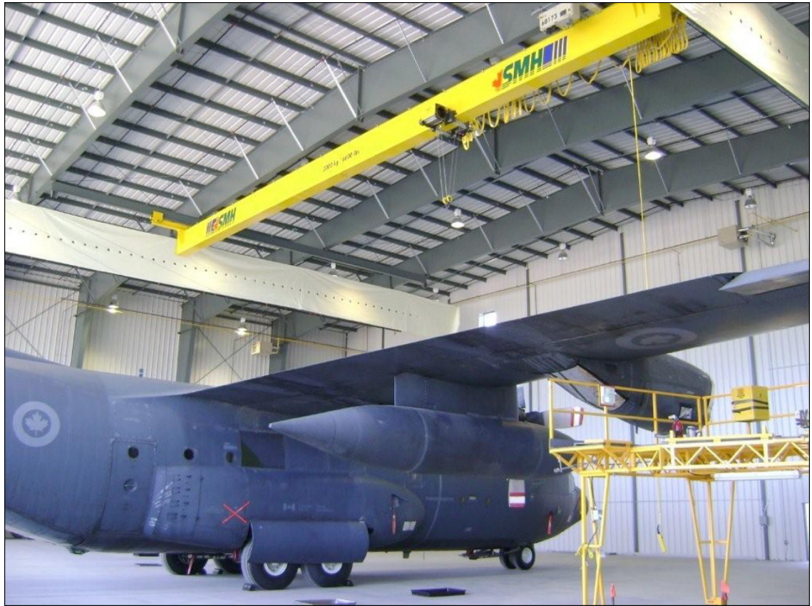
Figure 5-2: Under Hung Crane
