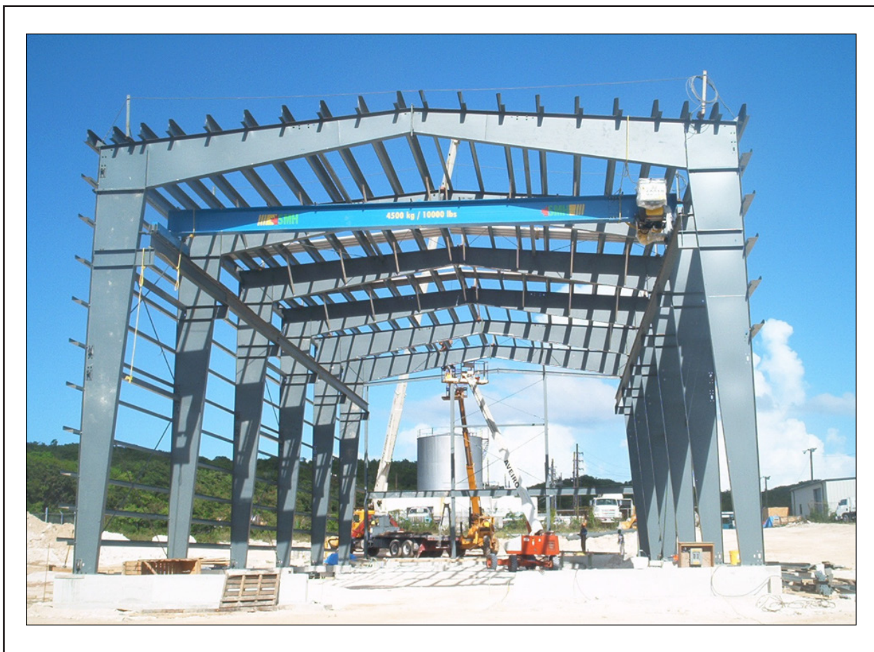
Figure 5-1: Top Running Crane
