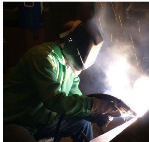
Certified welder adding metal accessories to primary structural steel frame.
