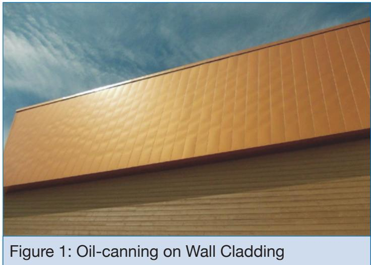
Figure 1: Oil-canning on Wall Cladding
