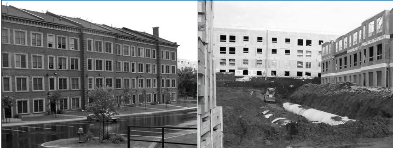
Figure 5: Corrugated steel pipe detention systems are unobtrusive and are sized to suit the site requirements
