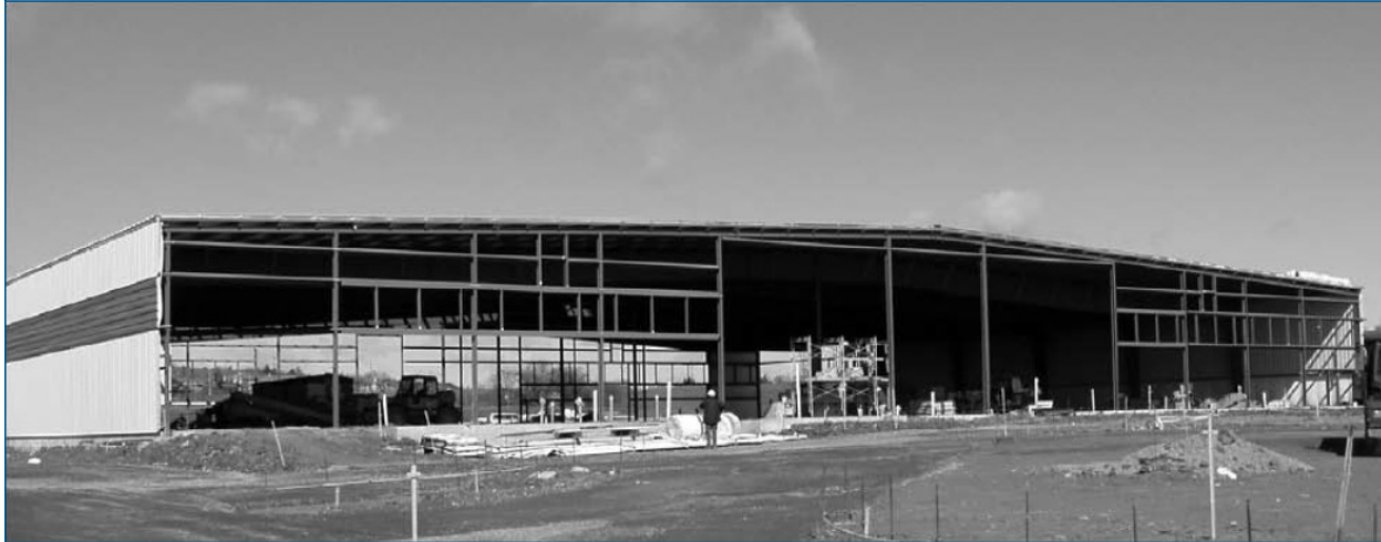
Figure 2: Typical sloped roof building site
