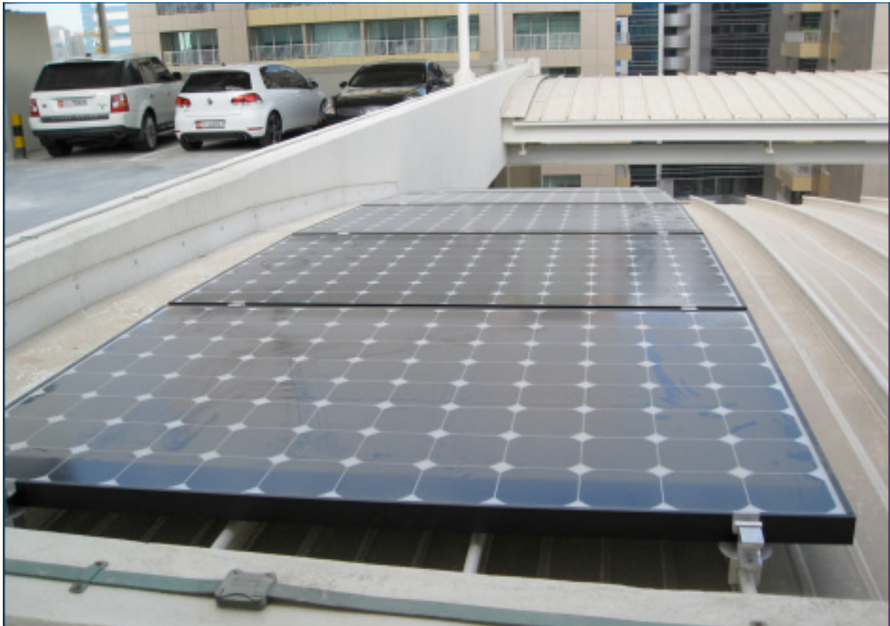
Figure 1: Solar Panel Installation on Steel Roof Panels
