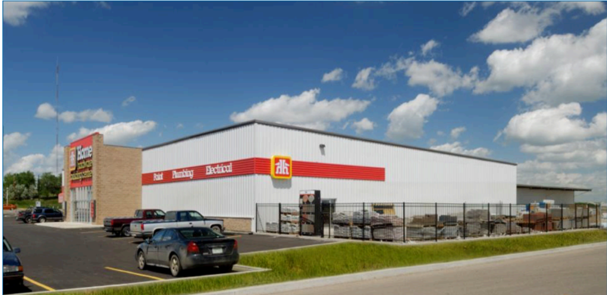
Figure 1: Retail Steel Building System
