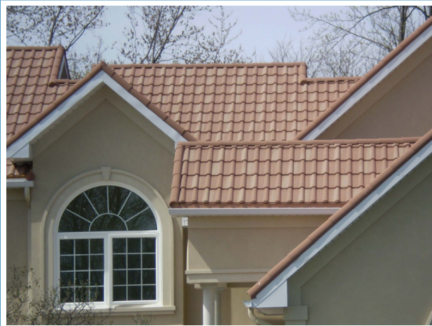
Example of steel-tile roofing profile.
