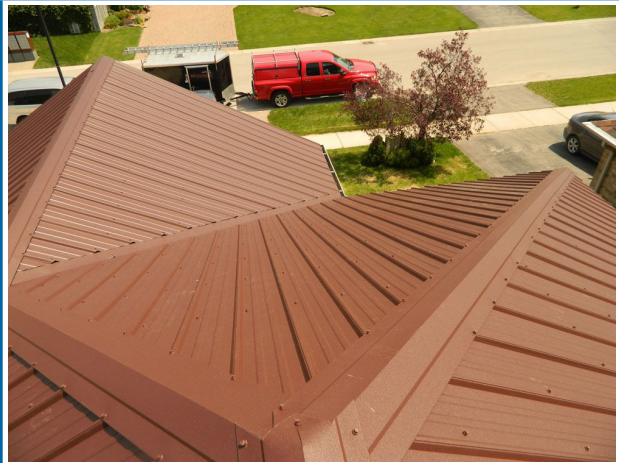
Example of vertical rib steel roofing profile.
