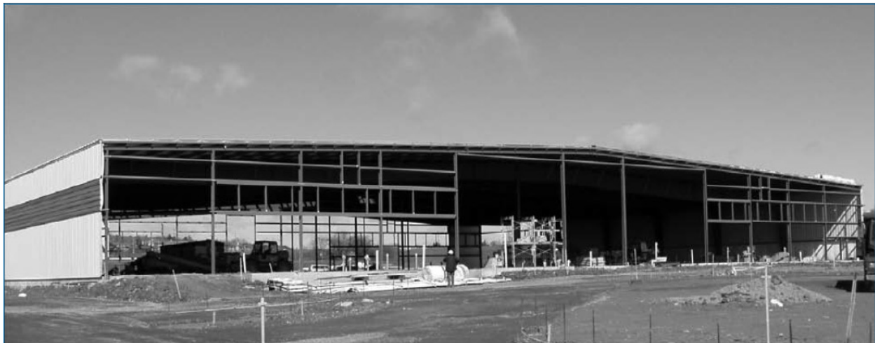
Figure 2: Typical sloped roof building site
