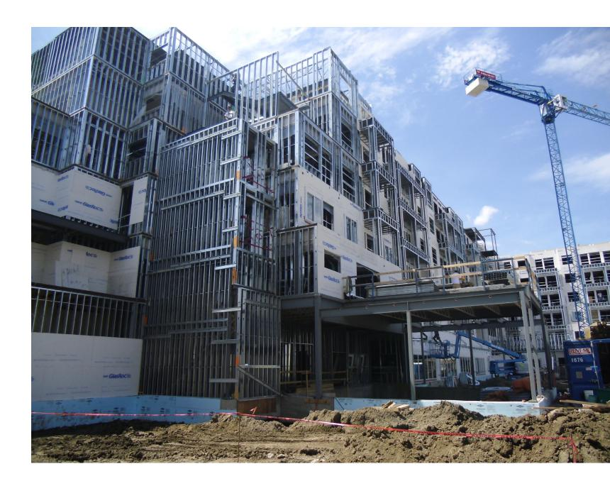
"We supplied all the cold formed steel and connectors. We had 95% pre-cut to size to save labour and site debris. The steel's precision and straightness allowed the use of pre-engineered panels. We estimate close to a \$10.00 per 0.093m<sup>2</sup> (\$10 per sq. ft.) savings over a concrete structure."
