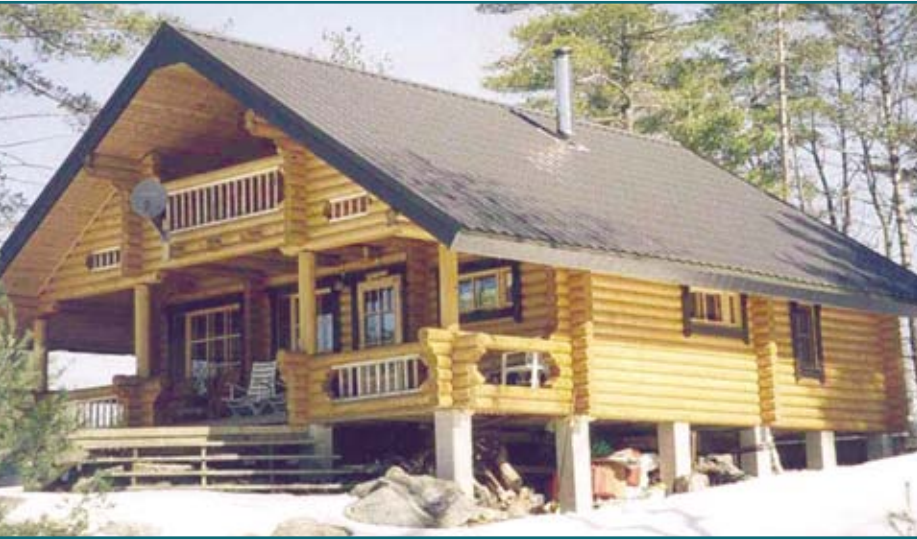
Figure 8: Ontario cottage, roof clad with Barrier 100/washcoat. Five years exposure.
