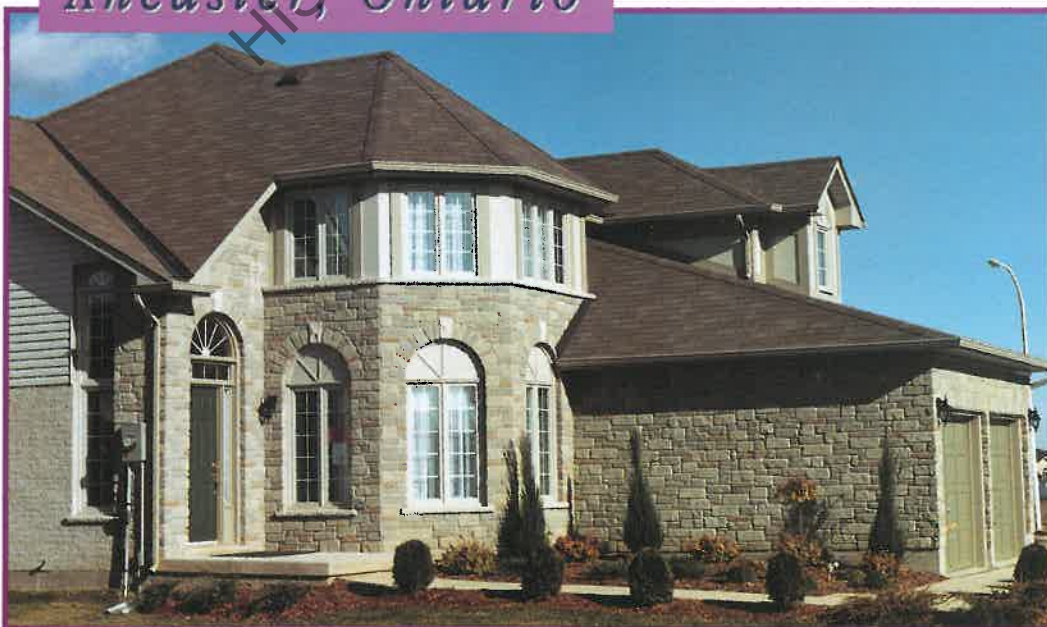
The first Homesteel project was built in Ancaster, Ontario. This home featured steel wall studs and floor joists in an otherwise traditional home.
