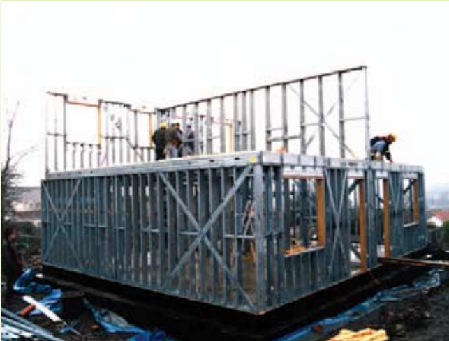
Figure 2 · Typical lightweight steel frame construction
