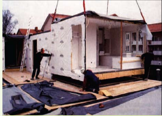
Figure 1 · Prefabrication can reduce impact of work on site
