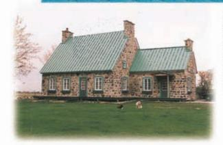
This type of roof is characterized by a linear shadow pattern which varies in the spacing and design. The ribs or standing seams can be flat and hidden or wide battens. Design and anchoring systems vary from one manufacturer to the other and the height, width and colour of these standing ribs will give each roof its own personality.
